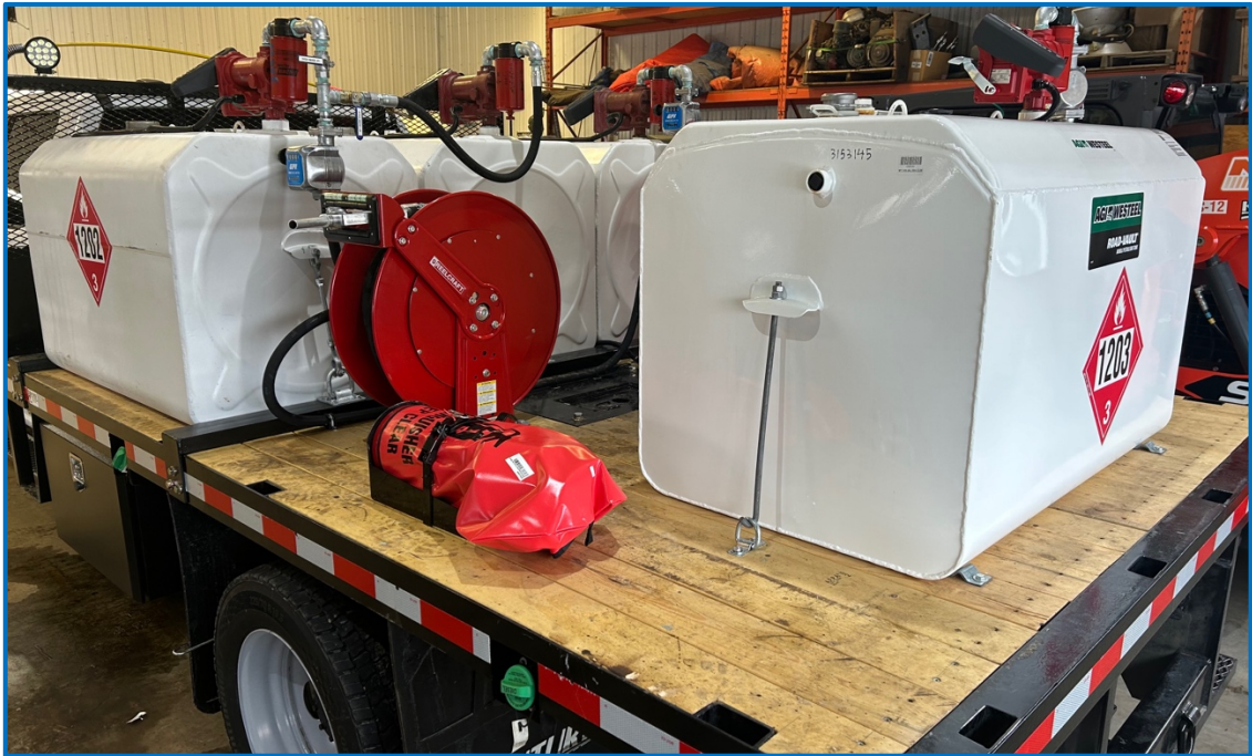
Image 3.0 - Image showing Gasoline Tank anchors and base supports
