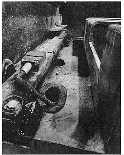
Tack welded the shuttle guides
