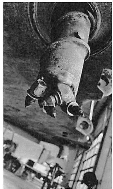
New carbide teeth installed on anchor
