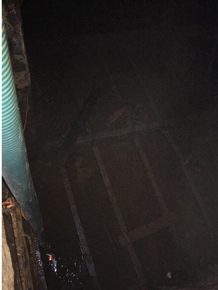
Figure 10 - View inside Void H
