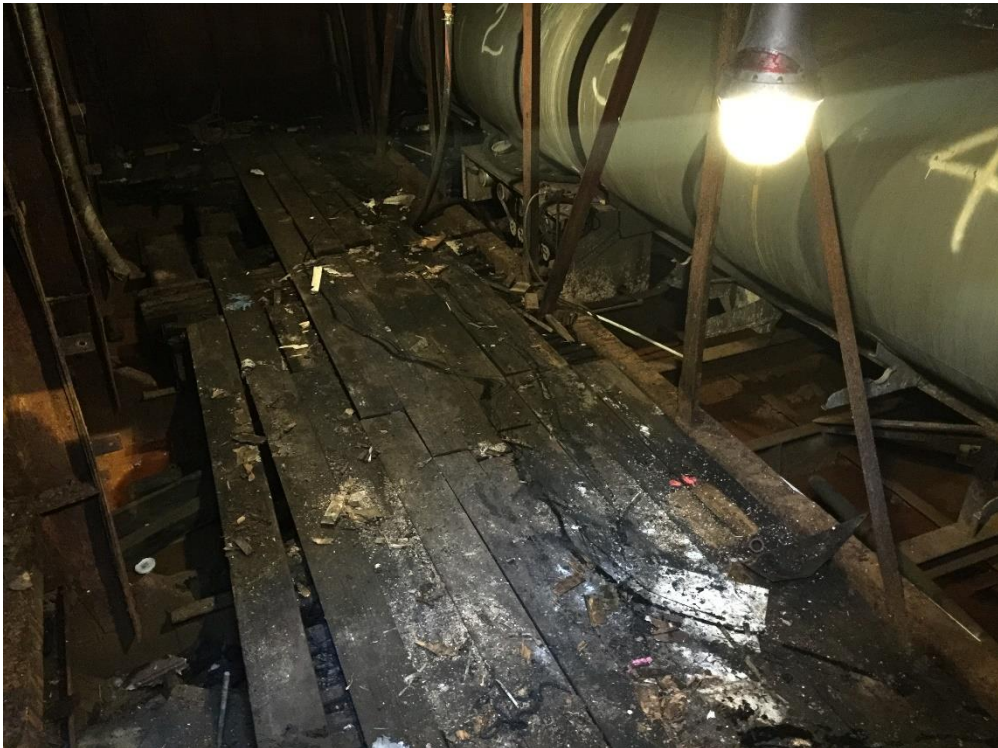
Figure 9 - View inside Void B, showing the aviation fuel dump tanks
