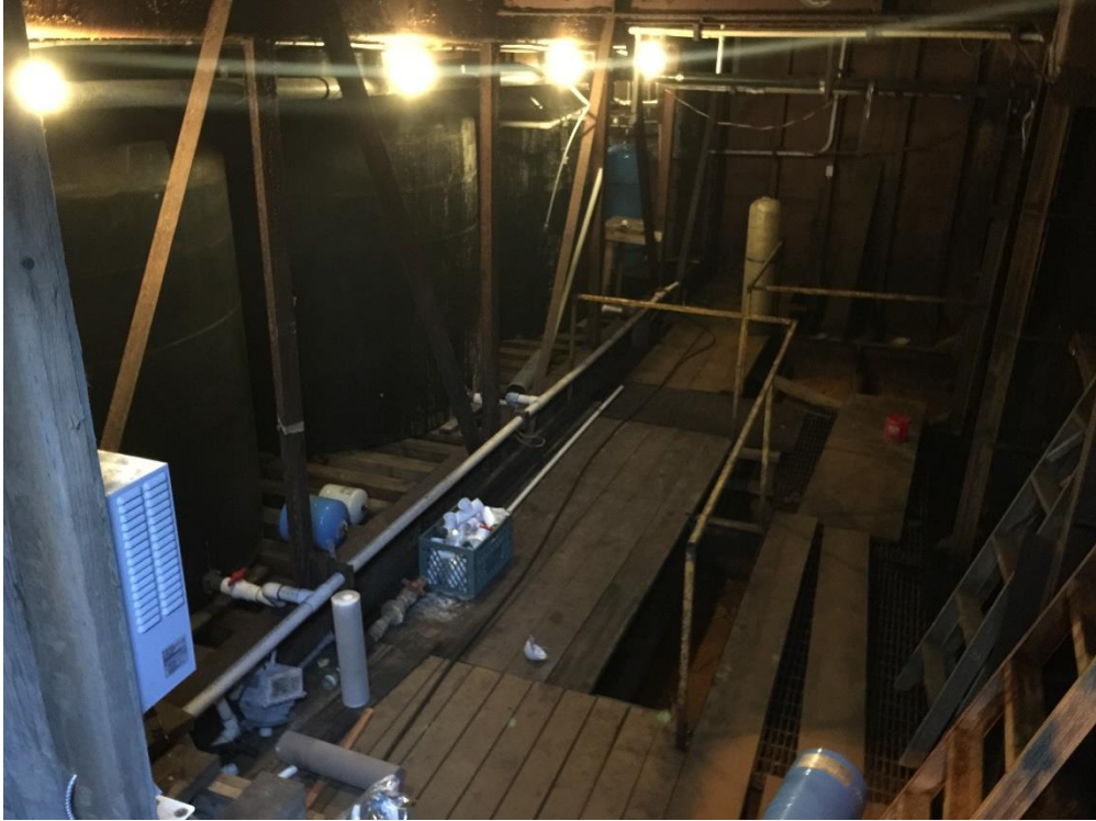
Figure 8 - View inside Void G, showing the FW tanks
