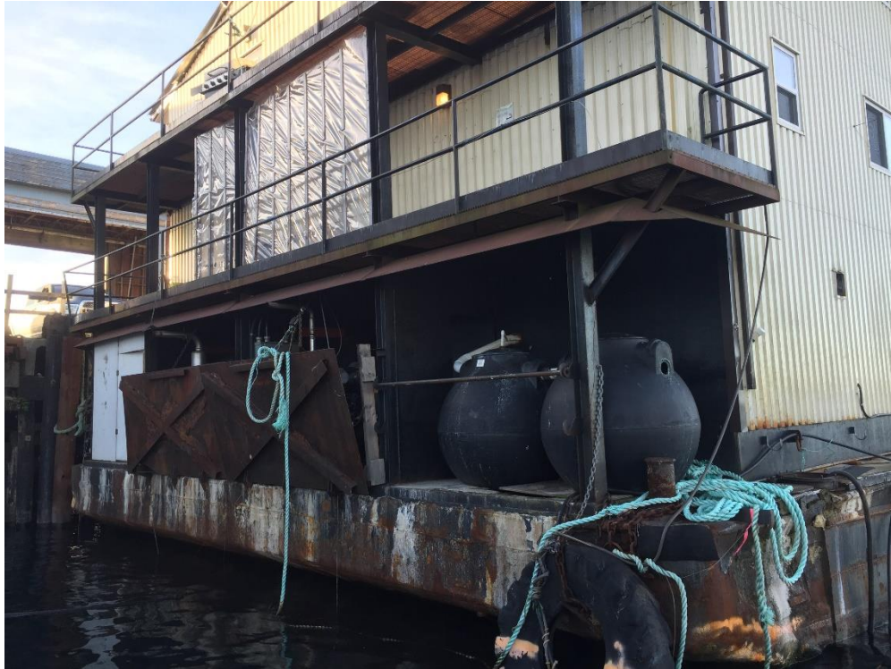
Figure 4 - View of the stern of the barge
