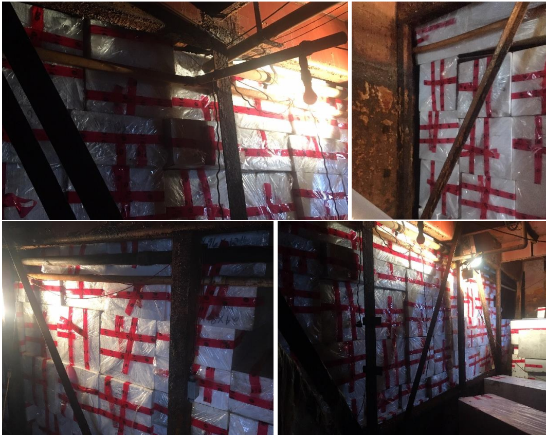
Figure 1 Foam block installation
