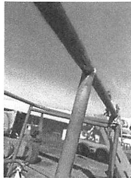
P9.11: Repair on Top Rail.
