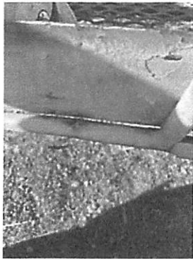
P9.10: Repair on Bottom Rail.
