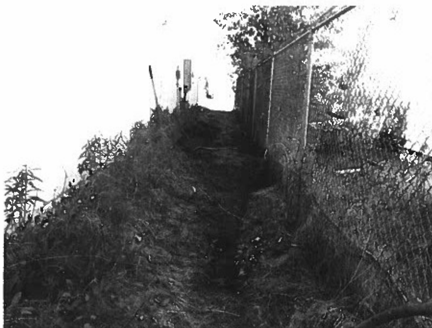
Photo 18: View of the excavation extent behind the building facing west.
