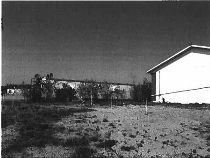
Photo 9: View of inside fenced yard immediately west of the site building.
