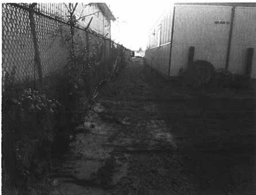
Photo 34: View of after backfilling behind the east trailer.
