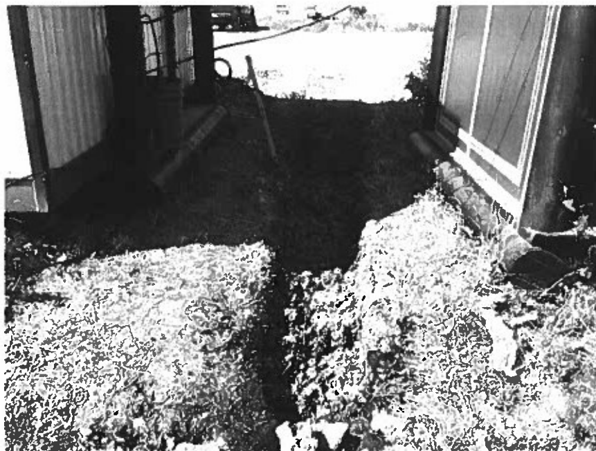
Photo 28: View of excavation in between the trailers.
