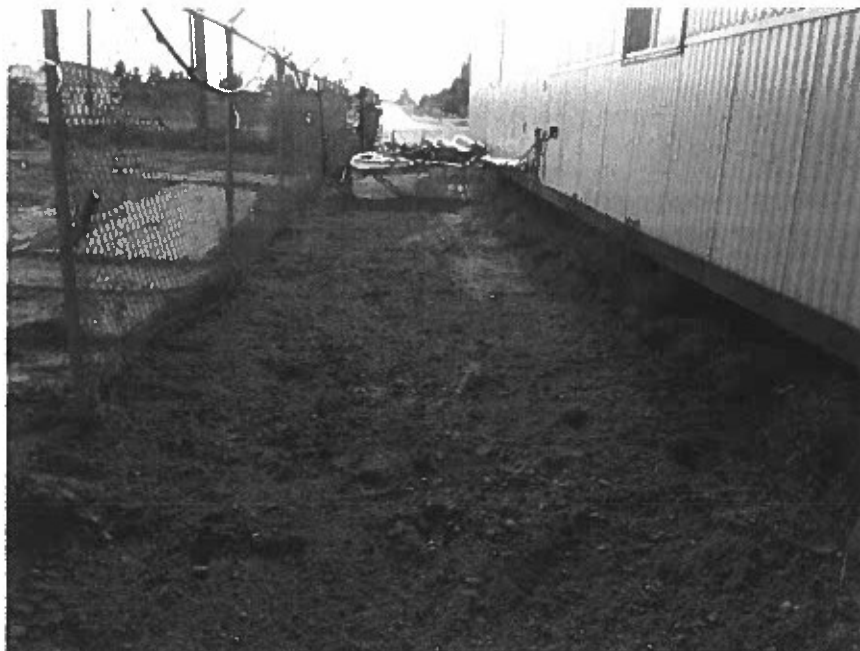
Photo 33: View of after backfilling behind the west trailer.
