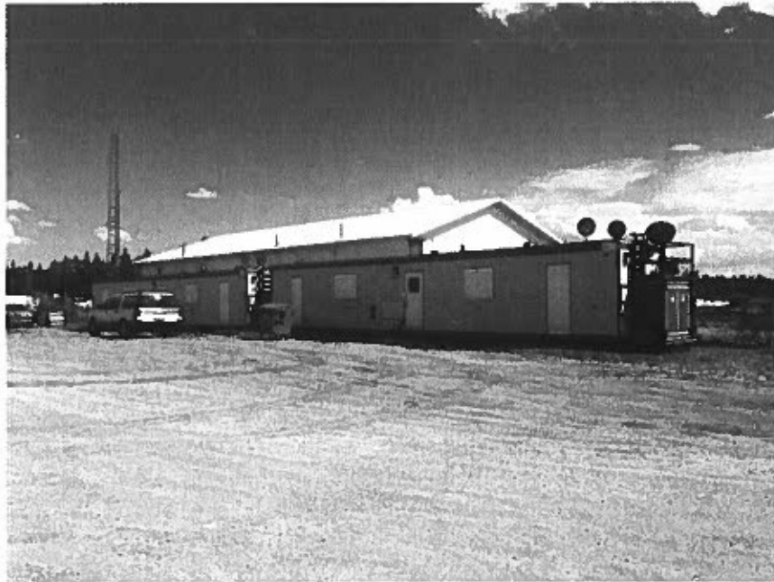
Photo 23: View of office/staff trailers facing southeast from the north adjacent property.
