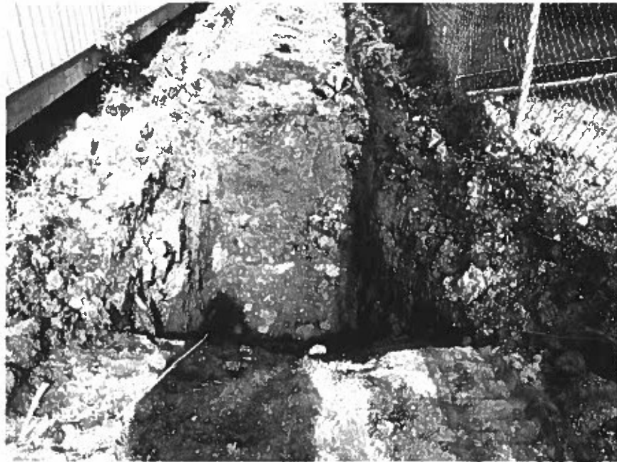
Photo 31: View of the deep excavation at JU34 location.
