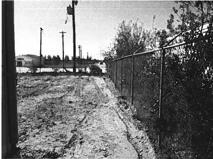
Photo 19: View of the yard after backfilling facing west
