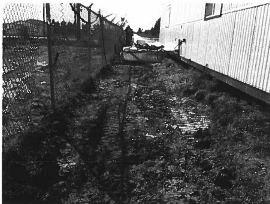
Photo 29: View of excavation behind the west trailer.
