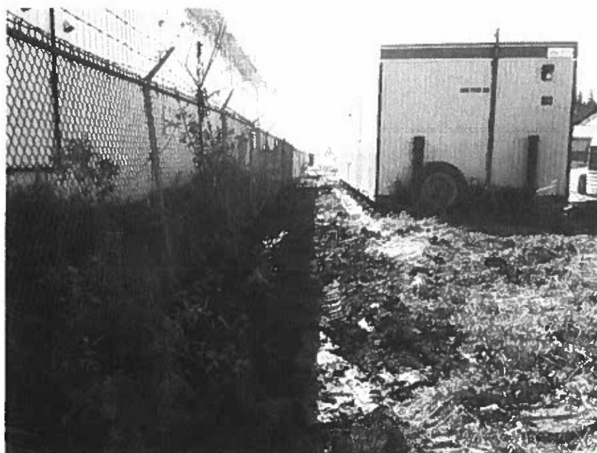
Photo 30: View of excavation behind the east trailer.
