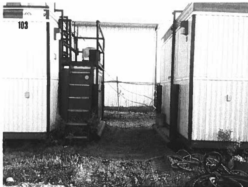
Photo 32: View of after backfilling between the trailers.
