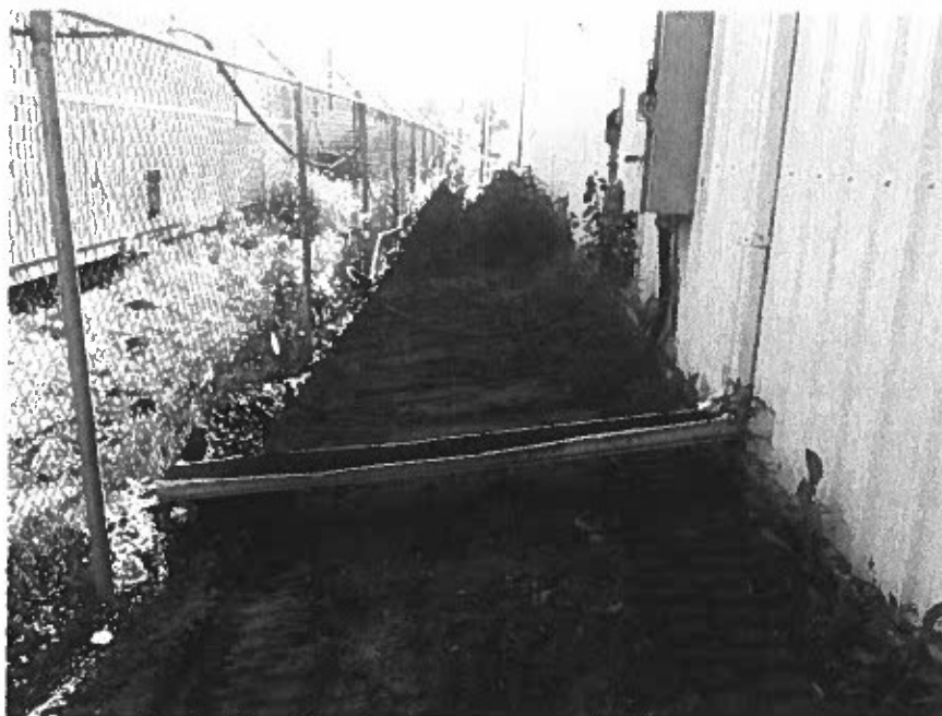
Photo 22: View of after backfilling at JU9 location.
