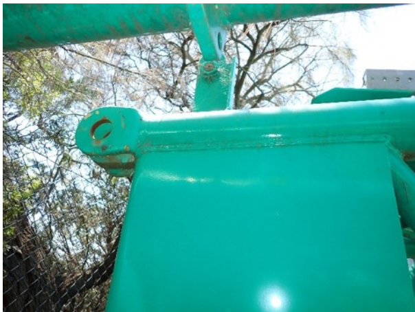
Connection end & lacing
