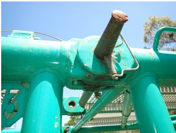
Connect end & lacing
