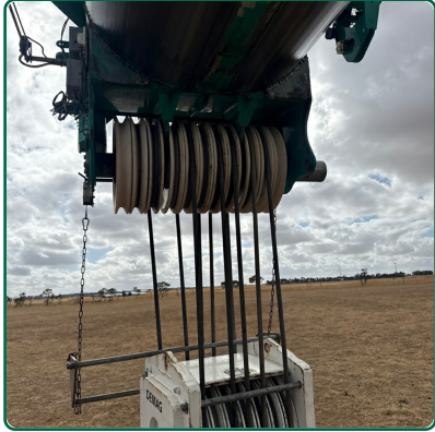
Head Sheaves and bearings
