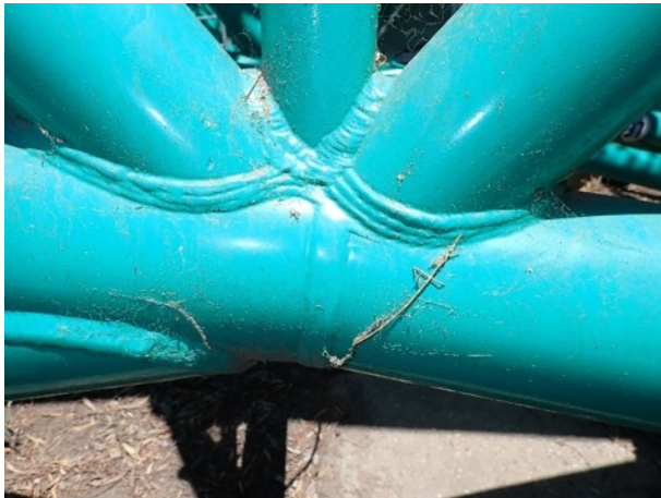
Butt weld & lacing
