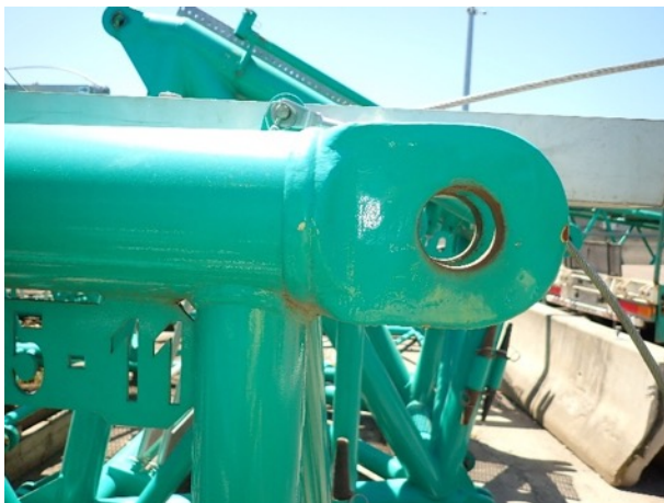
Connection end & lacing
