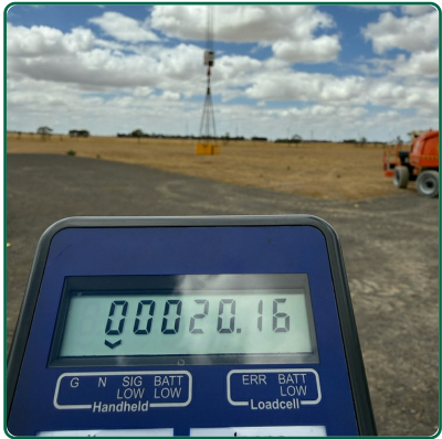
Rated Capacity Limiter Fitted 2060kg+hook block and rigging motion cut as per the load chart
