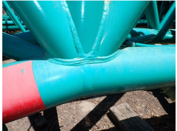
Butt weld & lacings
