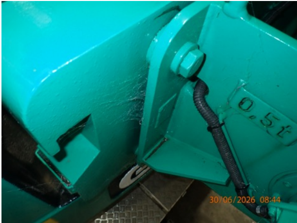
Photo 9: Winch mount welds
