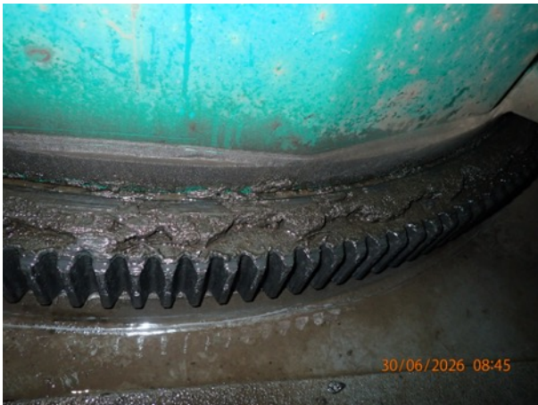
Photo 5: Outer slew bolts
