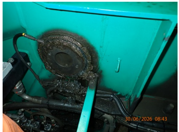
Photo 12: Butt pinning hole weld
