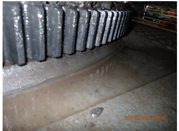
Photo 4: Slew ring weld
