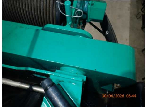
Photo 10: Winch mount welds
