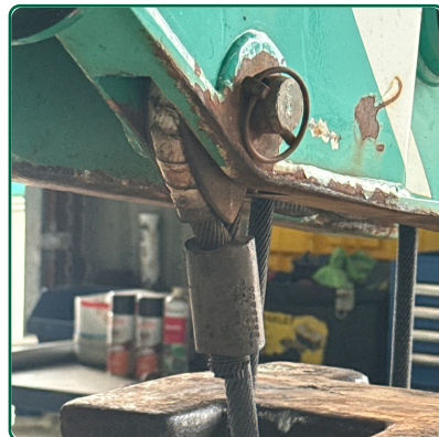
Main Hoist Rope Socket and Pins
