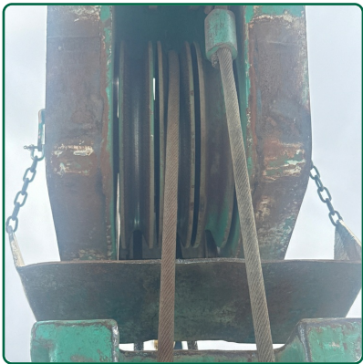
Head Sheaves and bearings
