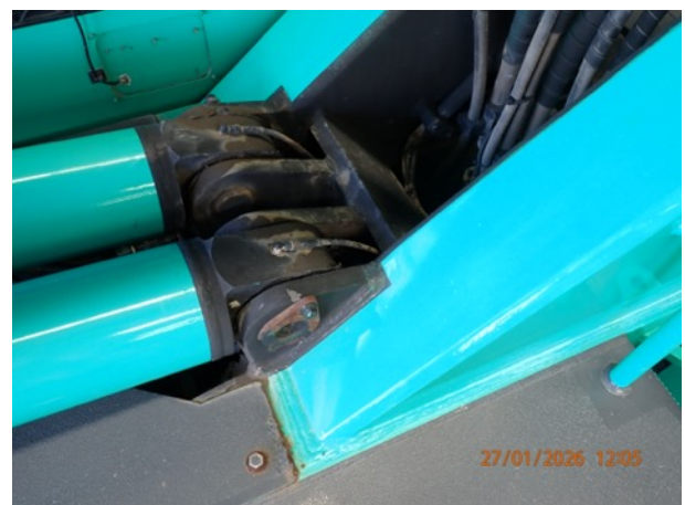
Photo 4: Lower luffing cylinder weld & mount
