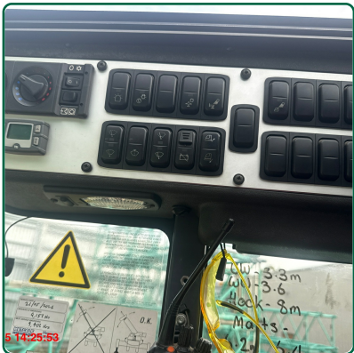
Switches and Relays
