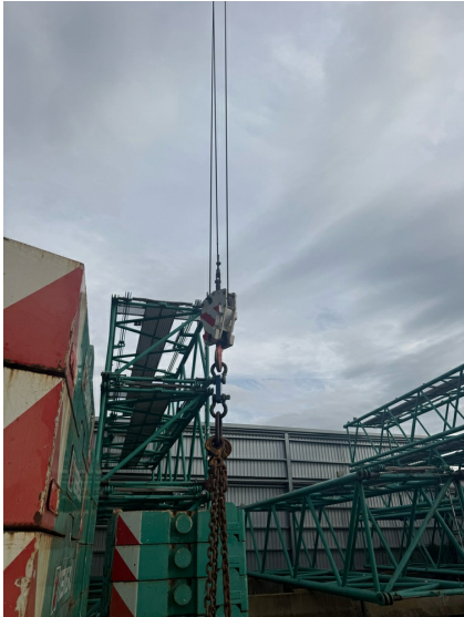
Line Pull Test
