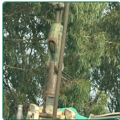
Main Hoist Rope Socket and Pins
