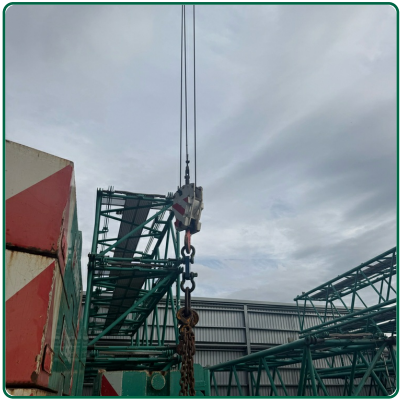
Line Pull Test
