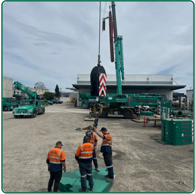
Line Pull Test
