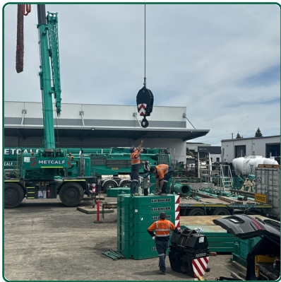
Line Pull Test
