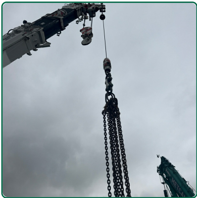
Line Pull Test
