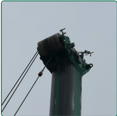
Idler Sheave and Bearing
