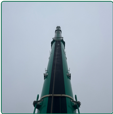
Shimming and Alignment
