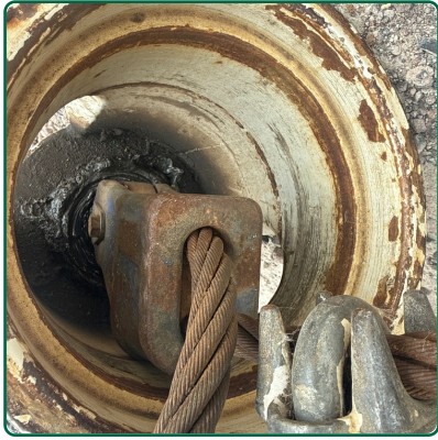
Auxiliary Hoist Rope Socket and Pins
