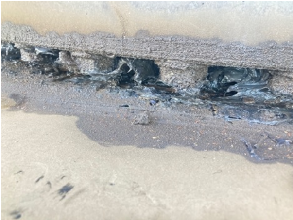
Photo 3: Slew ring weld
