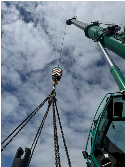
Line Pull Test
