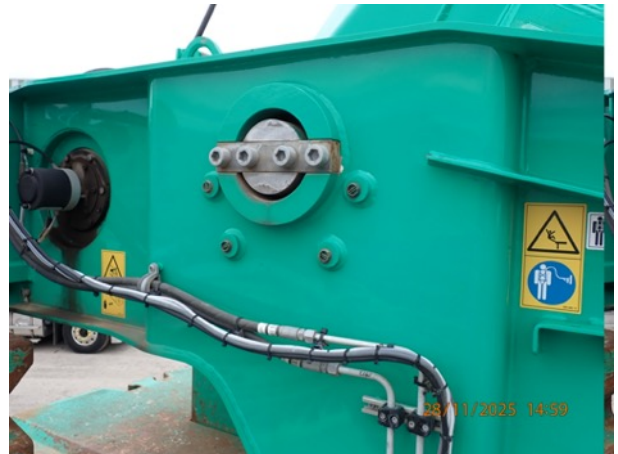
Photo 8: Turret & butt pinning hole weld
