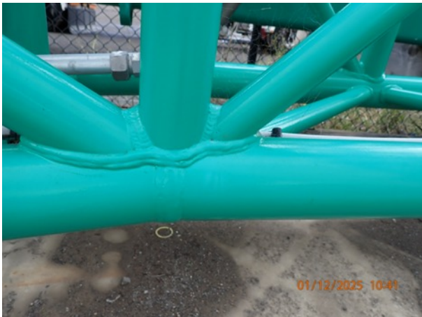
Photo 23: Fly butt weld & lacings
