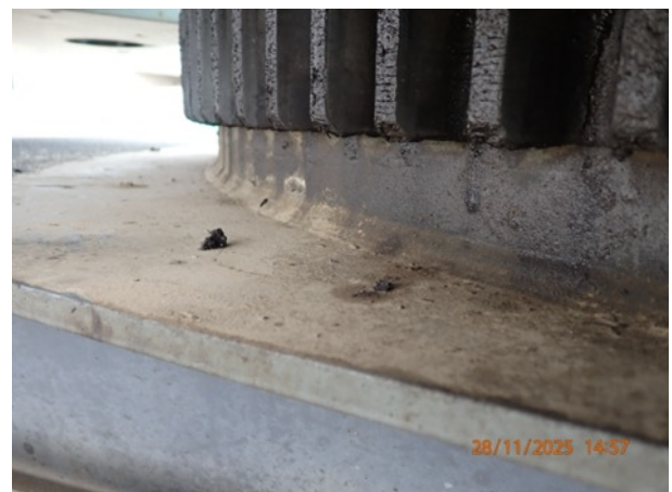
Photo 4: Slew ring weld
