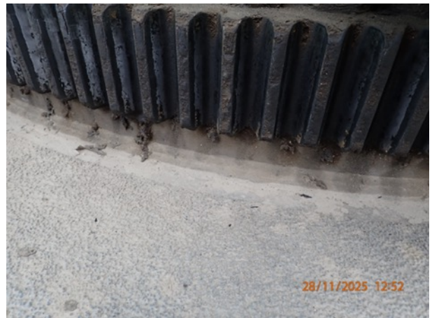
Photo 4: Slew ring weld
