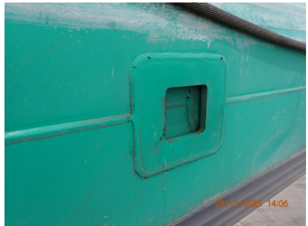
Photo 12: Boom pinning hole welds
